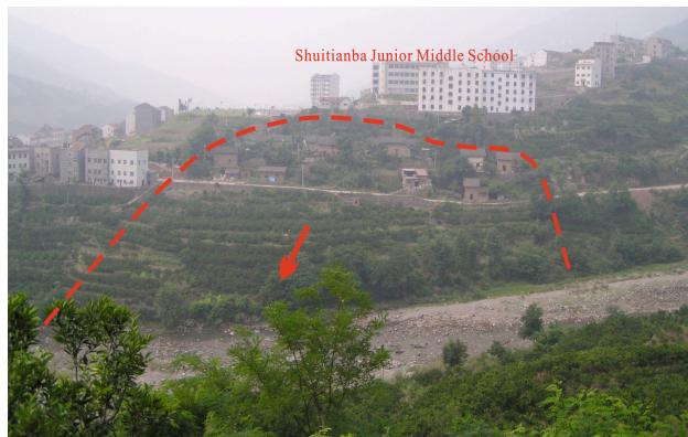
Fig. 8. View of the Xiatudiling landslide
