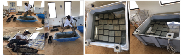
Fig. 4. Concrete mixing and Curing.
