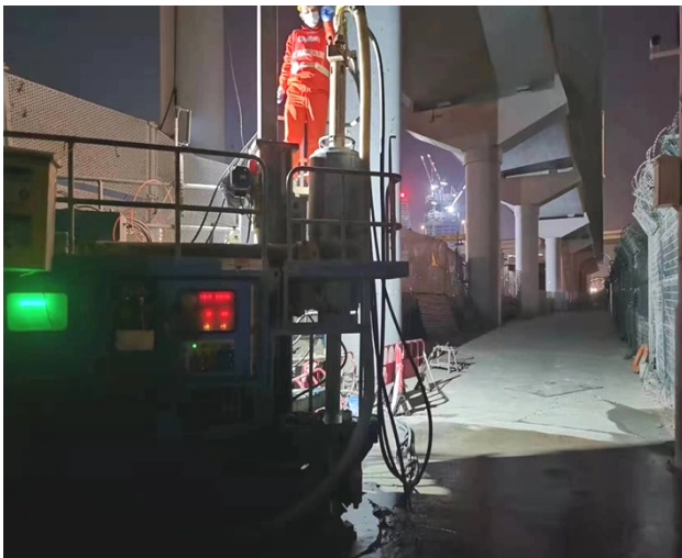
Fig. 4. Construction site of MJS pile.
