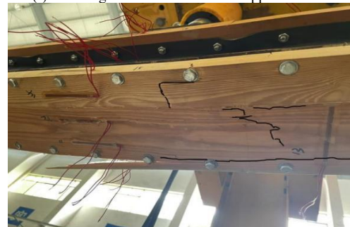
(g) Parallel-to-grain tensile cracking of timber on beam L2 bottom plate
