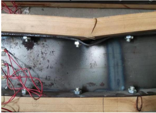
(i) Buckling of beam L2 steel web upper exterior
