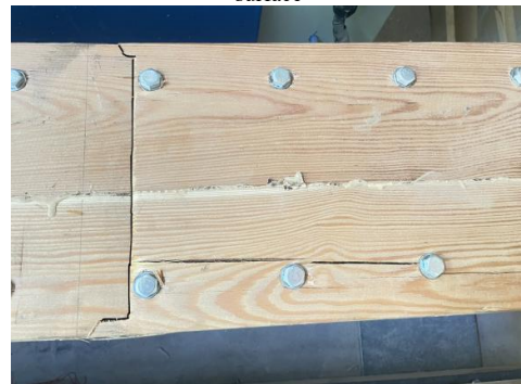
(e) Parallel-to-grain buckling and local splitting of timber on beam L1 top surface
