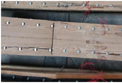
(h) Parallel-to-grain buckling and local splitting of timber on beam L2 top surface
