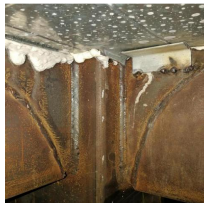
(b) Inner side of SJ-1 jointing weld
