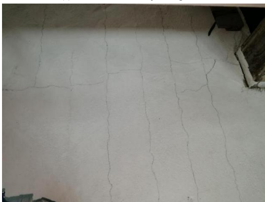
(c) SJ-2 crack picture
