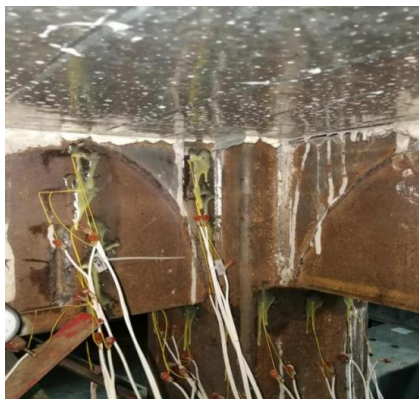
(a) Outer side of SJ-2 jointing weld
