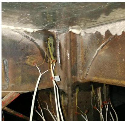
(a) Outer side of SJ-1 jointing weld
