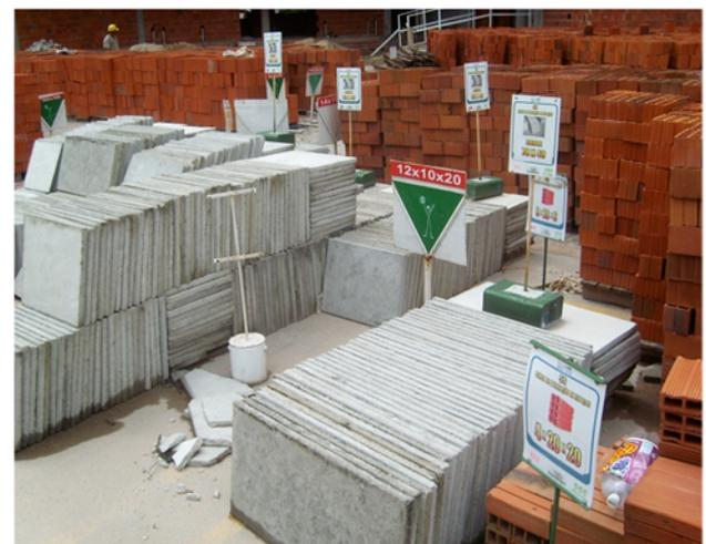
**Fig. 8.** Organization of construction sites based on visual Management and 5S
